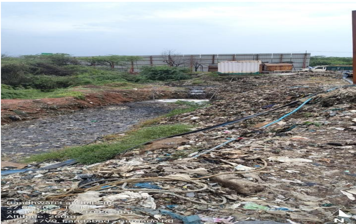
Kutcha drain carrying leachate to adjacent plantation area
