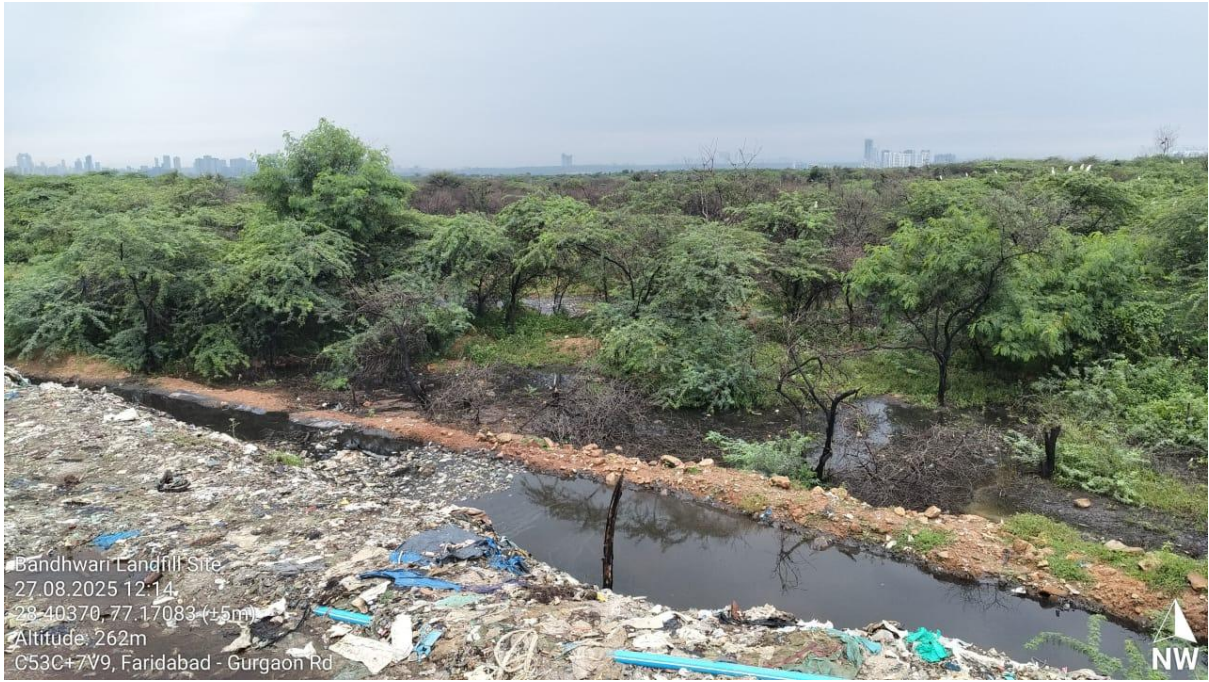
Kutcha drain carrying leachate to adjacent plantation area
