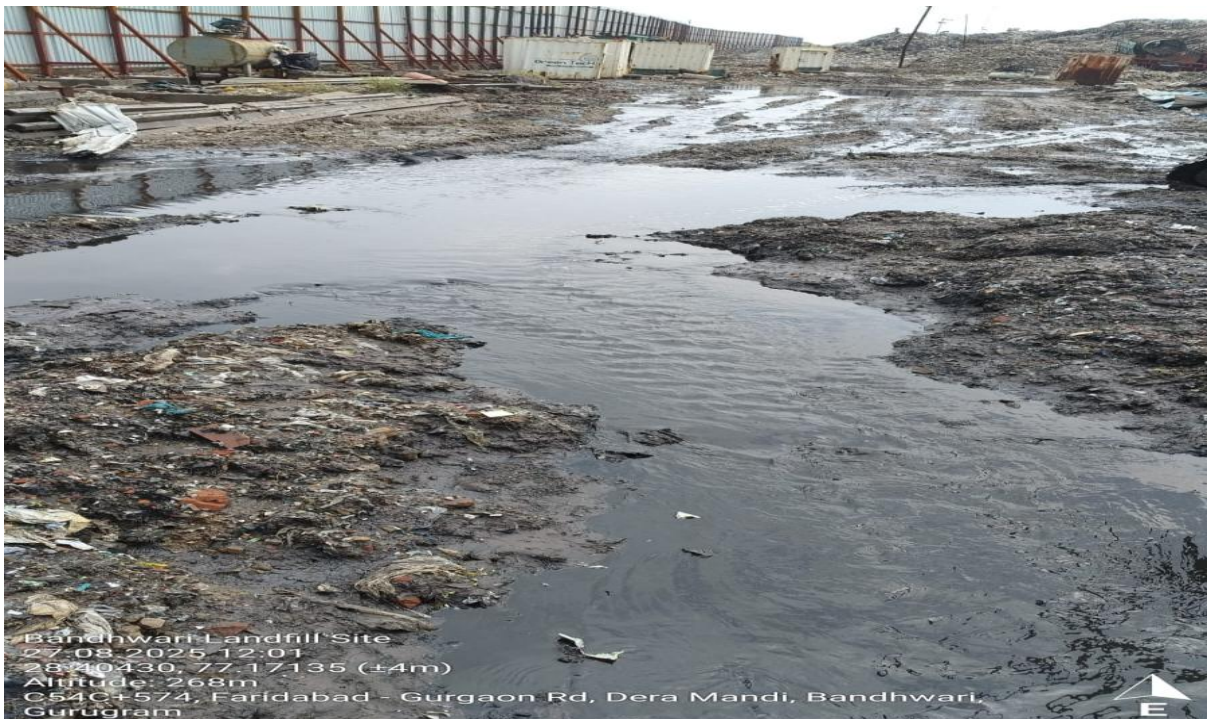
Overflowing of Leachate at Site
