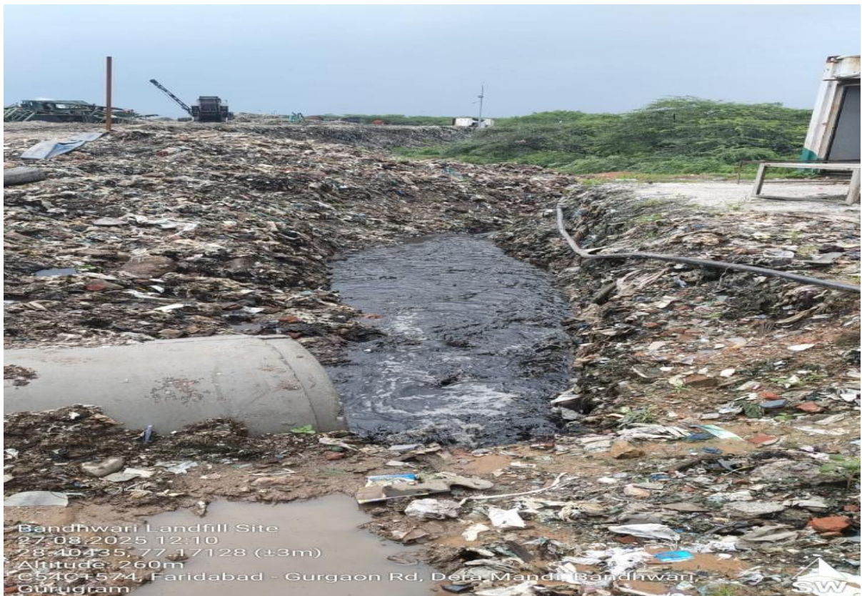
Diversion of leachate through concrete pipe
