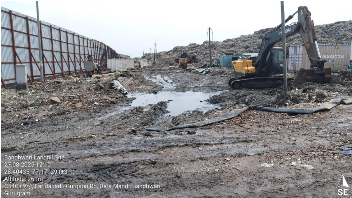
Overflowing of Leachate at Site
